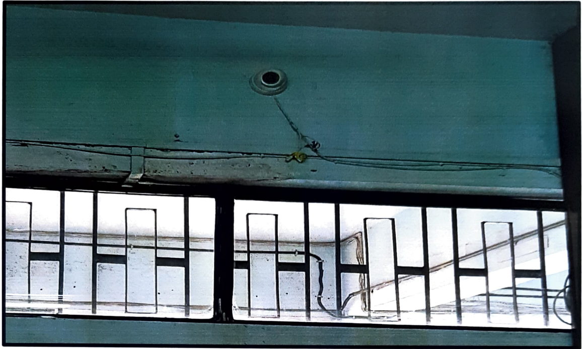
Closed circuit Cameras in every classroom, staffroom, office, library etc
