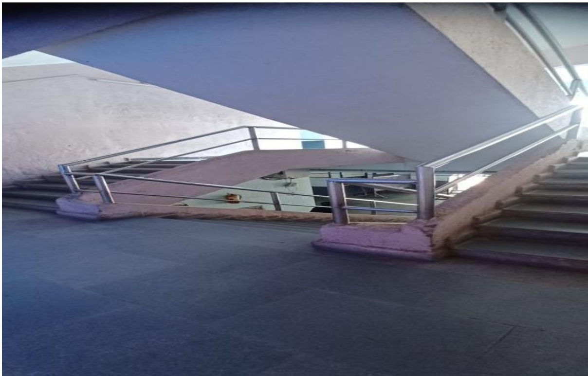
Railing at Staircase
