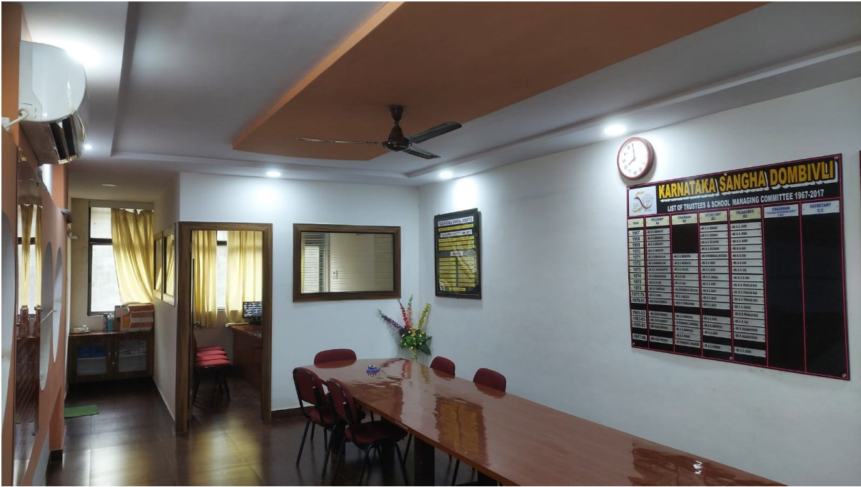
Use of LED in Management Room
